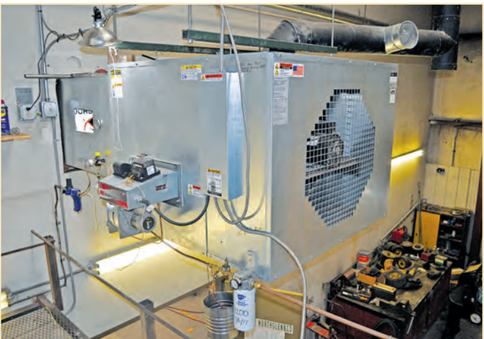
Motor oil heater at the fleet maintenance shop.
